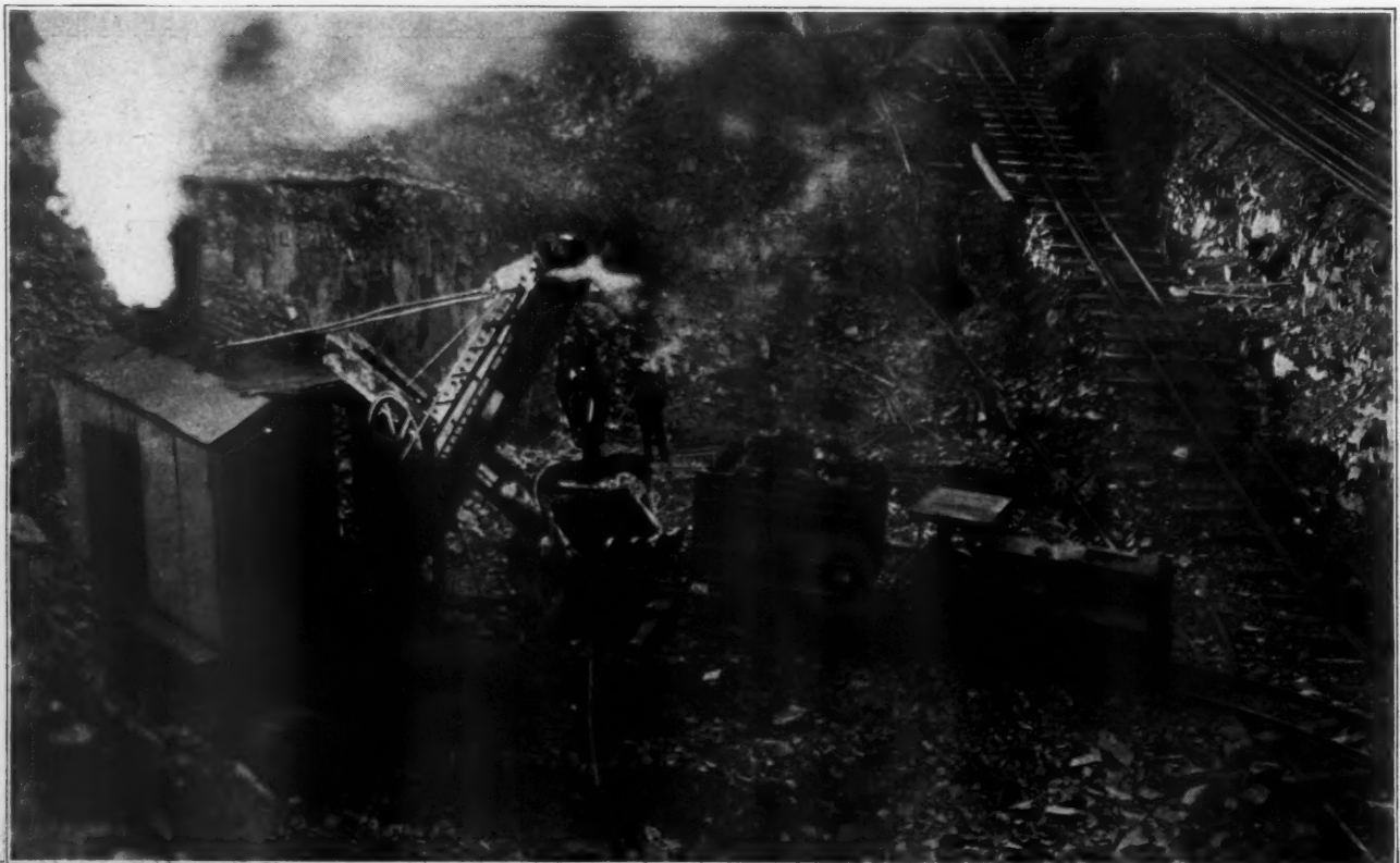
Shovel Loading at New Lower Level. Note the incline to Primary Crusher. The old incline from the Upper Level is at the right.
